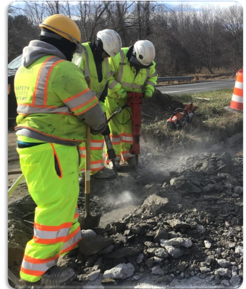
Crew removing Raised Median
