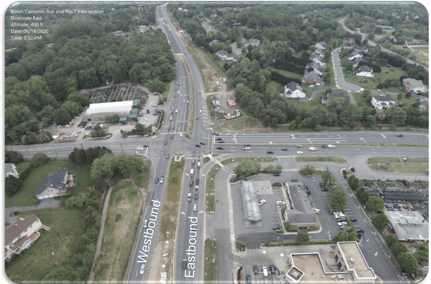
Route 7 Baron/Cameron Avenue Looking East
